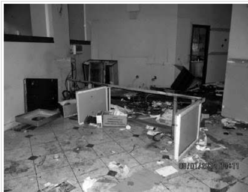
Figure 6 K*VOX before repairs
